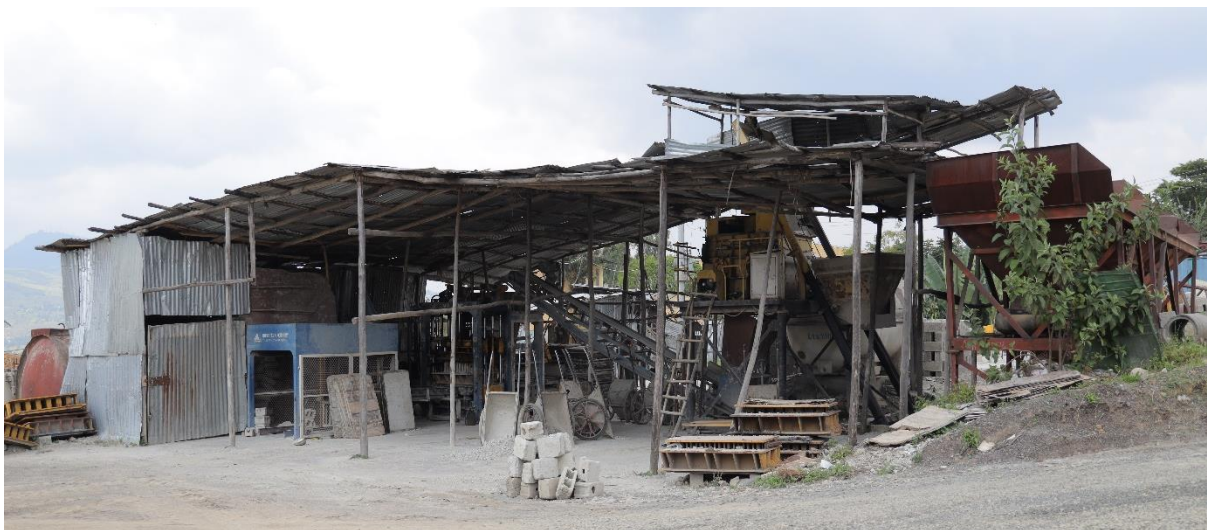
HCB Production Plant
